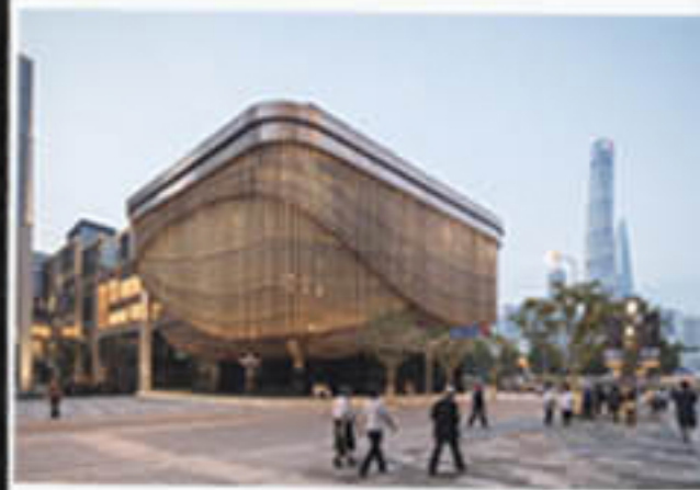
The Bund Finance Center is a building in The Bund, Shanghai, China. It is notable for its three, overlapping, moving layers of vertical stainless steel pipes. These layers, inspired by theatre curtains, slowly rotate around the building. Designed by Heatherwick studio and Foster studio
