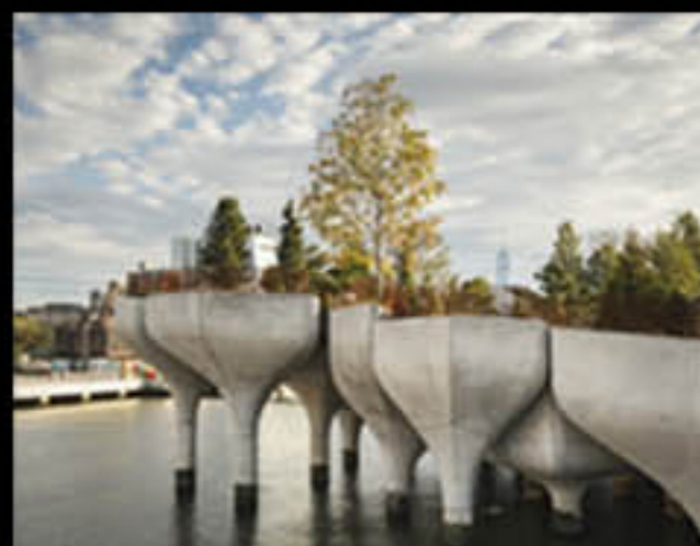
Little Island or Pier 56 Plans arose in November 2014 for a new park designed by Heatherwick Studio, with estimates of the 2.3-acre. The park will float completely above the river Hutsen, resting on 300 concrete pillars. Park will be finish in 2021.
